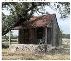
This 128 year old house is located about 4 miles north of Wimberley and was originally owned by W.H. and Liddie Dobie. It is board and batten construction built with no 2x4 studs. The chimney is made entirely with adobe. It wasn't until 1970 that the house was insulated, wired, and plumbed for an indoor bathroom.
